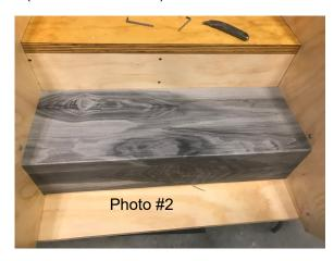
Fitting of preformed LVT "Six Degrees" step down riser treads, shown in Photo #2 leaves you a few options.
