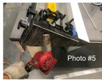
Photo #5 shows LVT preformed tread, on a site fabricated cutting block, being heated from below so cutting becomes quicker, using less effort.
